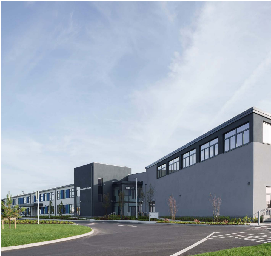
Mercy Secondary School, Kilbeggan, Co. Westmeath – completed project ADAPT 1.
