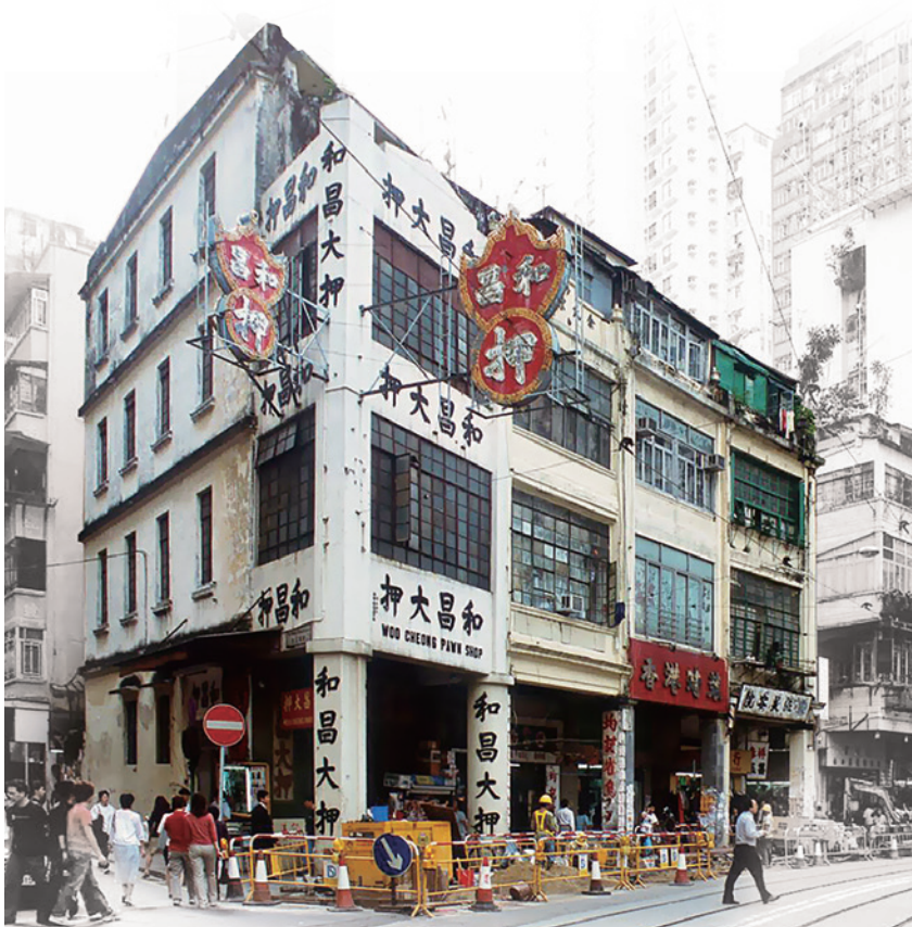
活化前的灣仔和昌大押，可見騎樓部分被業主圍封佔用。 Prior to revitalization, Woo Cheong Pawn Shop in Wan Chai had its overhanging balconies sealed by landlords.
