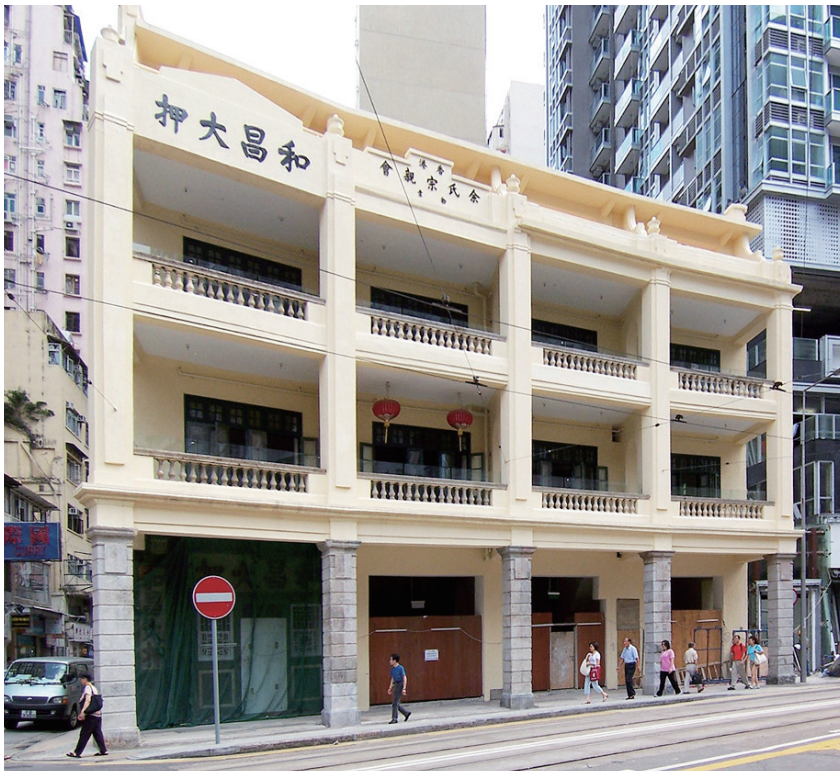
活化後的灣仔和昌大押，騎樓圍封的部分被拆除，回復本來面貌。 Woo Cheong Pawn Shop in Wan Chai: after revitalization, the sealing materials of overhanging balconies were removed, and the building's appearance is restored.
