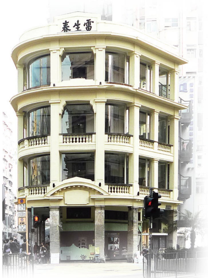
位於深水埗的雷生春，屬罕見的弧形轉角騎樓，現活化作中醫保健中心。 Lui Seng Chun in Sham Shui Po is a rare built structure that features curved-corner overhanging balconies. It now houses a Chinese medicine and healthcare center.
