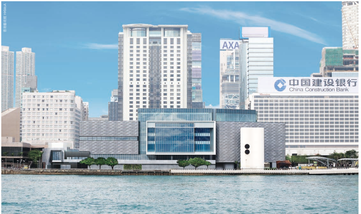
香港藝術館的外牆利用了立體纖維水泥板覆面模仿維港波浪的元素。 Façades of HKMoA with three-dimensional fibre cement board cladding simulate undulating waves of Victoria Harbor.
