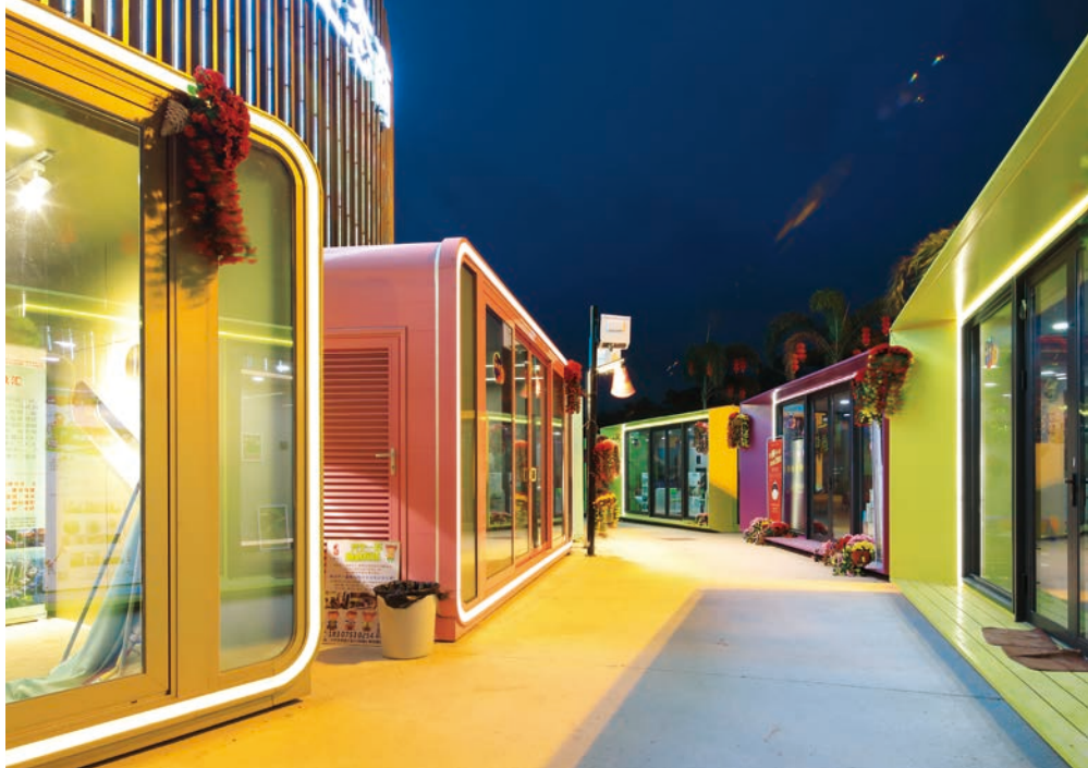
今年春節期間開幕的梅州興寧客天下商業街採用顏色繽紛的鋁合金組屋設置而成。 The Hakka Park commercial street in Xingning, Meizhou, opened during Lunar New Year, was built with a colorful array of aluminum alloy modular houses.
