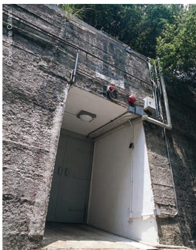
部分舊軍火庫地堡被保留。 Part of the bunker is preserved.
